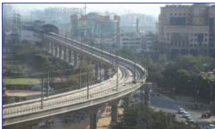
DMRC constructs sharpest curve in Gurgaon
