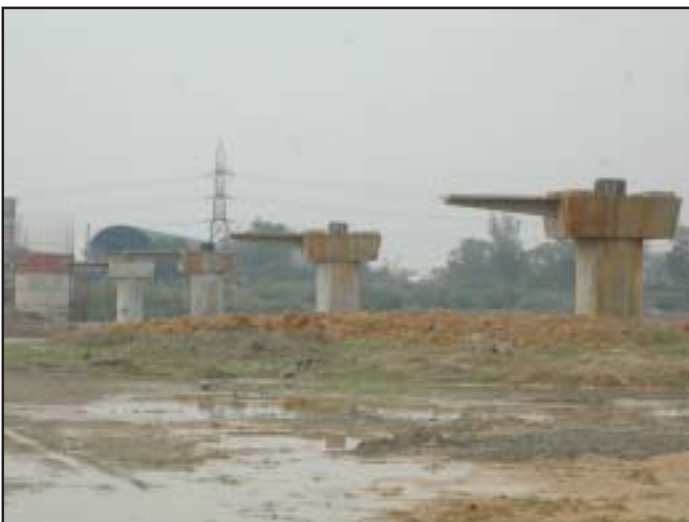
Yamuna bridge under construction
