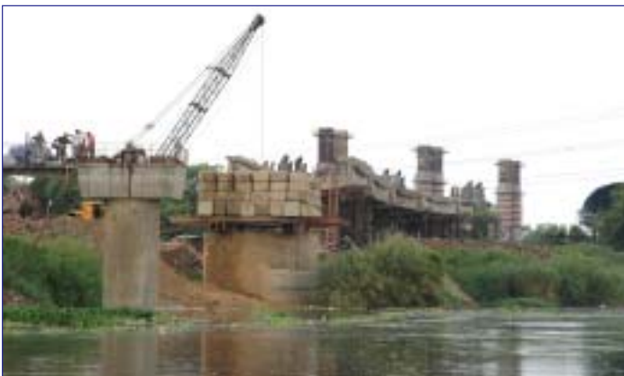
New Yamuna Bridge under construction
