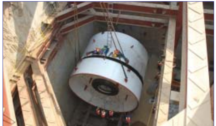
Tunnel Boring Machine in action
