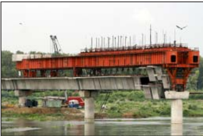
Construction work in progress
